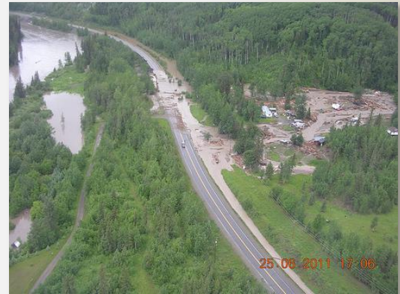
Fur Thief Creek Culvert (Pine Pass)
