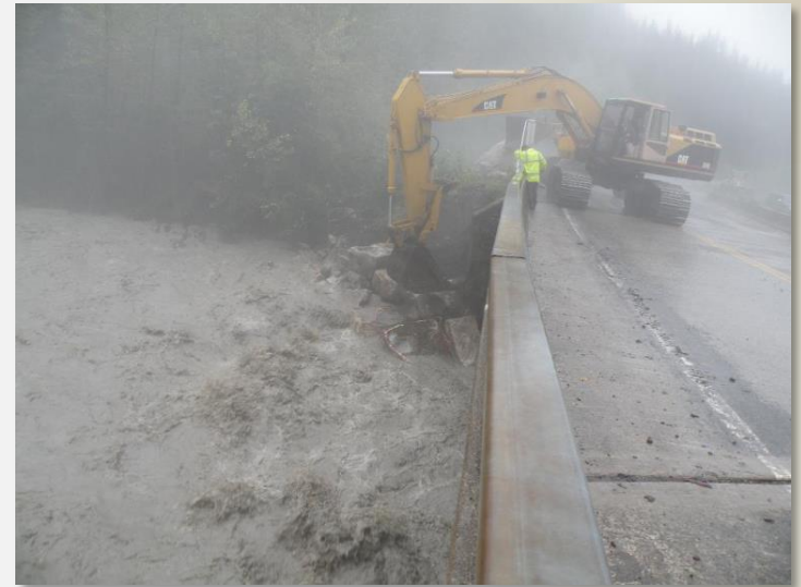
Bitter Creek Bridge (Stewart, Sept 2011)
