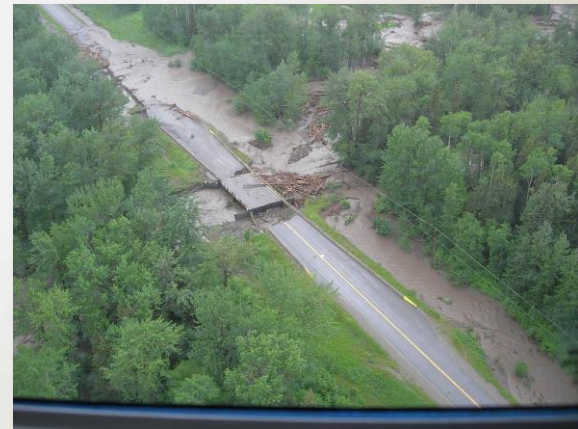
Fisher Creek Bridge (Pine Pass, June-July 2011)
